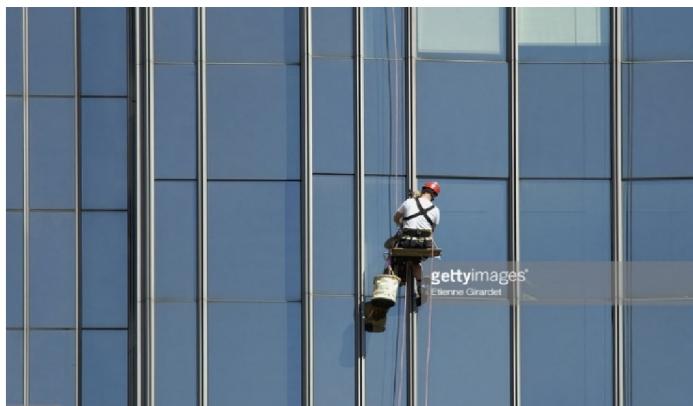
Fig 1 Manual Method of wall cleaning
