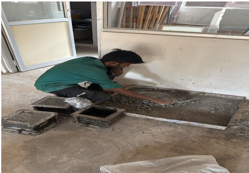
Fig 4: Preparing of Concrete and Casting
